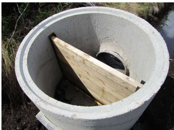
Reguliavimo šulinys. Foto: Airi Kulmala http://www.balticdeal.eu/wp-content/uploads/2011/06/2regulation_well1.jpg
